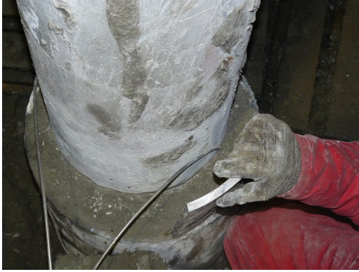
(a) Decentralized Anchor Casing in HE-53.
