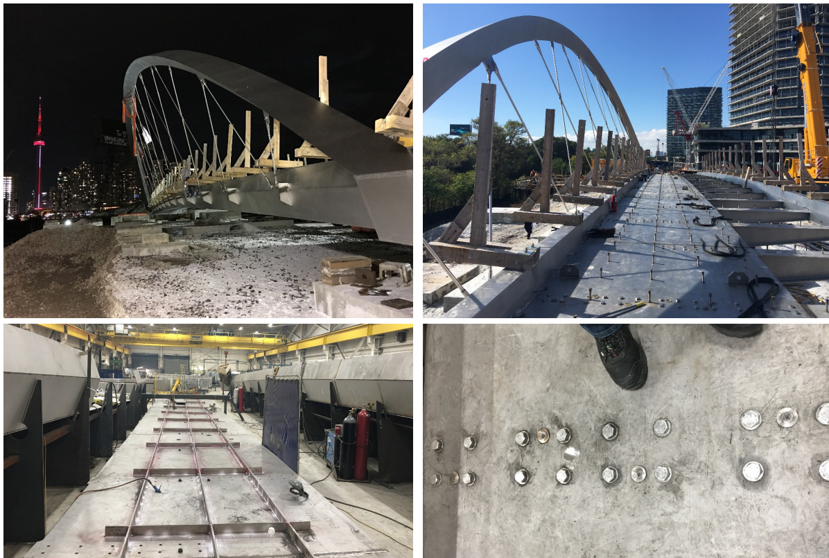
Figure 1-2: Garrison Crossing footbridge with slip-resistant connections made of stainless steel (Fort York Bridge, Toronto, Canada) © Juan A. Sobrino, pedelta
