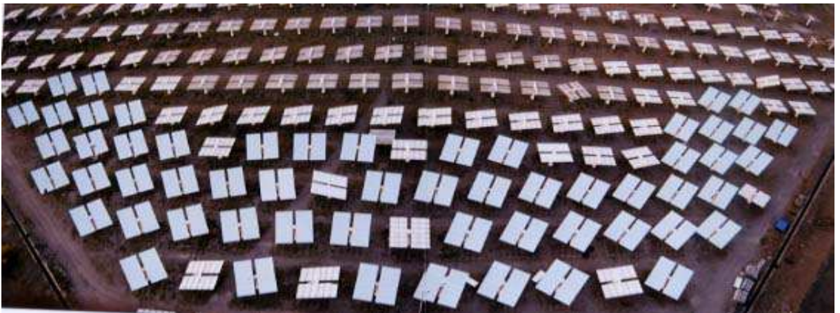
Figure 3.4: GRAAL heliostat field seen from above. The heliostats used by GRAAL are pointing to the tower (compare with the sketch of fig. 3.3).
