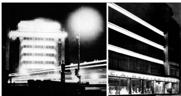
Fig. 2: Ely J. Kahn, Zimmermann Saxe and Zimmerman Associated, New York, 1919 (left), Erich Mendelsohn, C. A. Herpich Sons, Furriers, Berlin, view by night (right)
