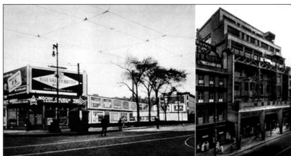
Fig. 3: New Street, Detroit, c. 1923–24 (left), Erich Mendelsohn, C. A. Herpich Sons, Furriers, Berlin, construction scaffolding (right)
