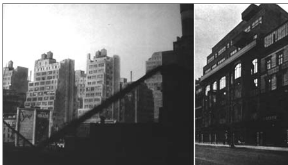
Fig. 4: View from a terrace of the Pennsylvania-Hotel, New York, 1924 (left), Erich Mendelsohn, C. A. Herpich Sons, Furriers, Berlin, view before facade refurbishment, 1926 (right)
