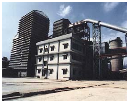
The Penden Cement Factory, opened in 1980, is fitted with filters to prevent air pollution.
