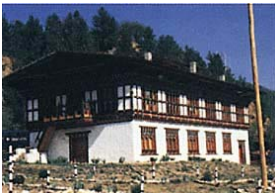
Within this structure build in the traditional Bhutanese style, research for the Renewable Natural Resources Sector is conducted.
