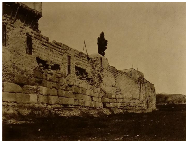
Figure 11: Watzinger and Wulzinger stated in the subtitle: “Arab City Wall with antique ashlar in L 4” (Watzinger/Wulzinger 1921, 58, fig. 35).
