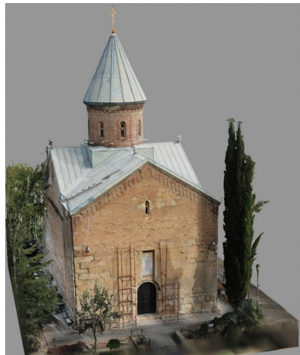
Figure 12. Meshed complete model with RealityCapture 1.0.3
