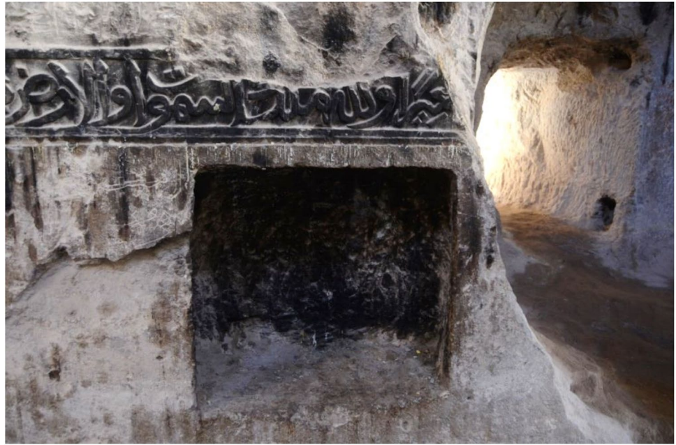
Fig. 3 Western wall of the rectangular hall in which the inscription has been damaged to create space E. Sockets to hold a wooden door are seen at the right corner of the portal
