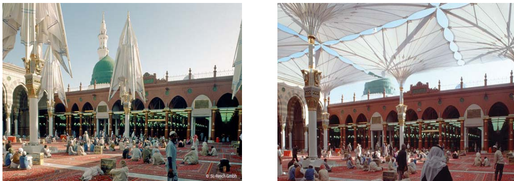
Figure 79. Umbrellas implemented in the Courtyard of the Prophet's Mosque in Madinah
