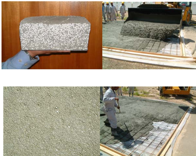
Figure 88. cross-section view of the final concrete/foam bubbles surface and the light-weight structure during production
